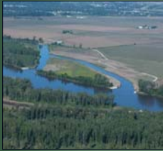
California Bend Chute – Chute Construction North of Blair, Nebraska
